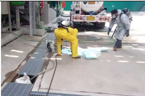
Picture 6. ERT used absorbance to cleanup spilled area and separate contaminate waste to hazardous waste disposal.
