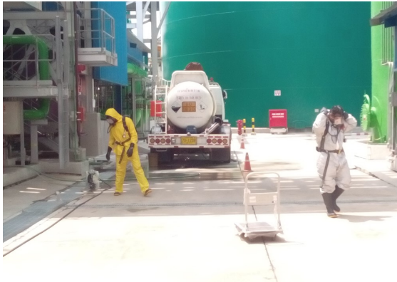
Picture 5. ERT used diaphragm pump transfer H 2 SO 4 to chemical pit and neutralization pit
