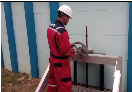
Picture 3. close sluice gate
