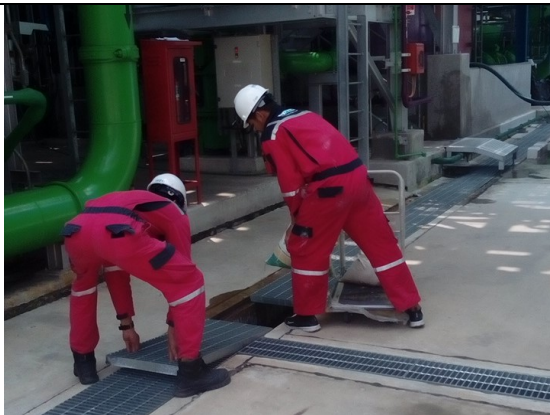
Picture 2. Field operator and helper used sand bag for block storm drainage
